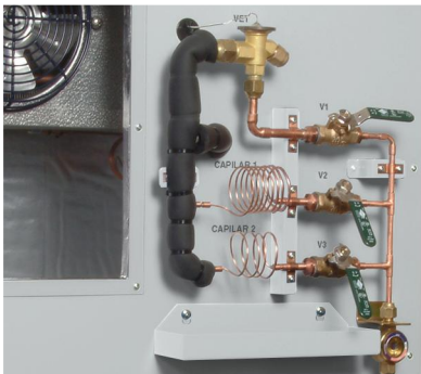
Figure 1. Three expansion (metering) devices are available.
